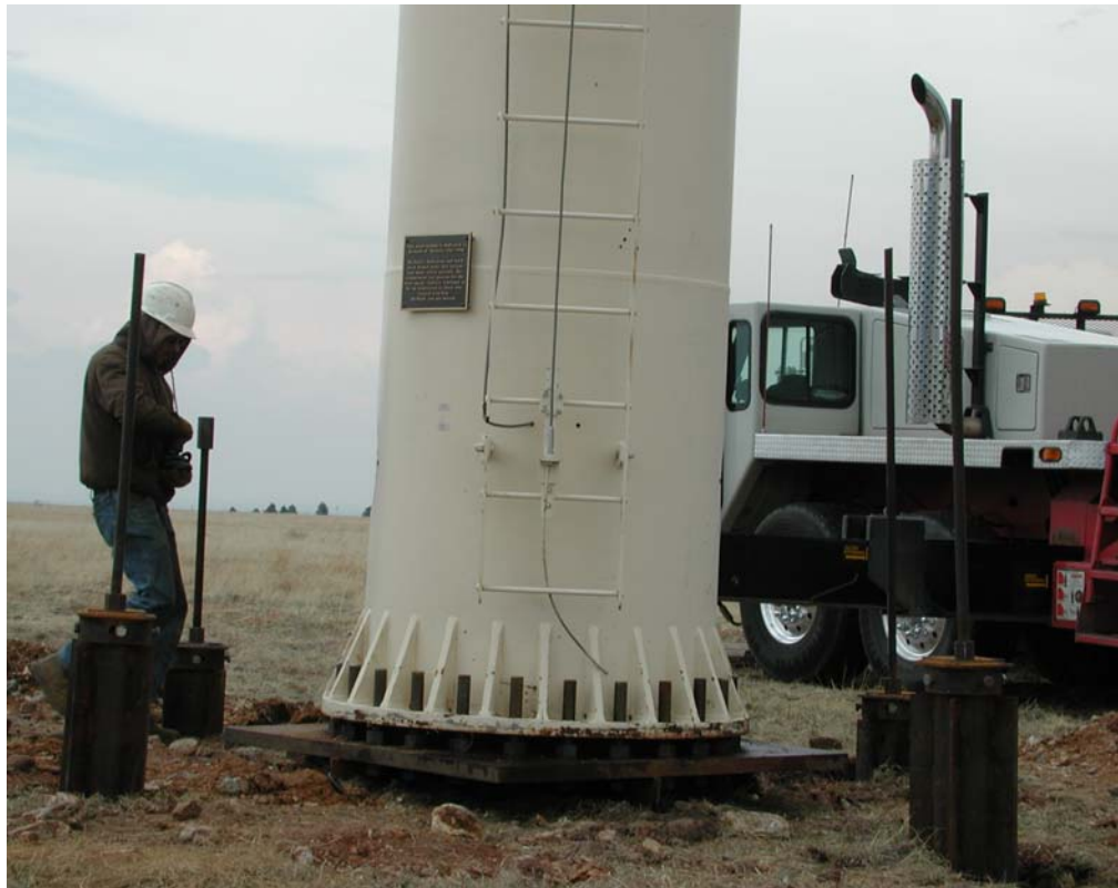
Figure 9: Photograph of the Moment Foundation After Tower Installation.
