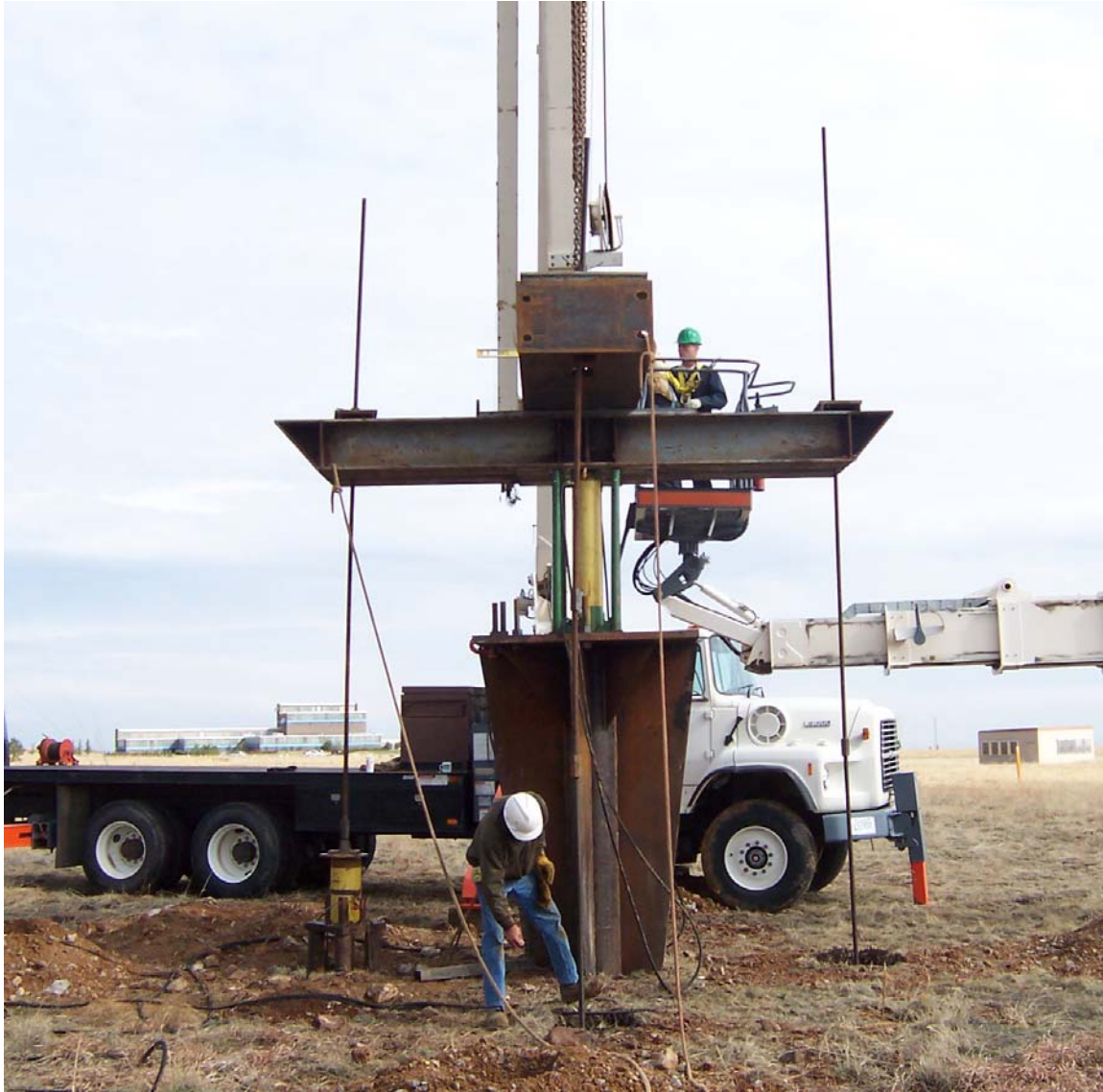
Figure 5: Photograph of the Moment Foundation Installation.
