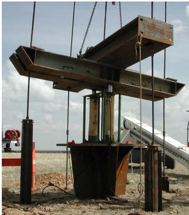
Figure 7: Photograph of the Stopping Point of the First Moment Foundation Installation Attempt.
