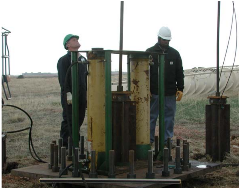
Figure 8: Photograph of the Moment Foundation After Successful Installation.
