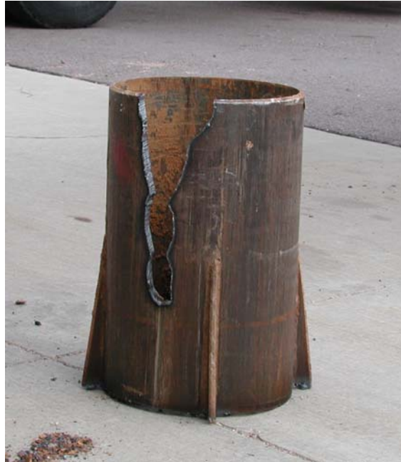
Figure 6: Photograph of the Moment Foundation Nose after Repair.
