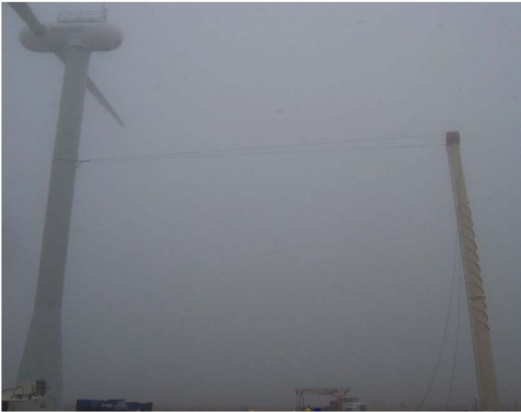
Figure 11: Tower Pull during Snow and Rain Storm
